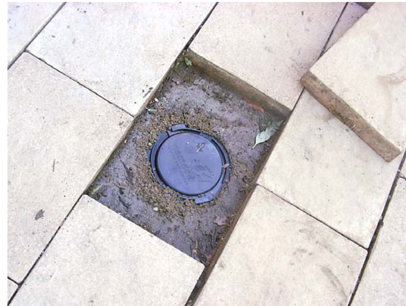
Inground Station installation directly under pavers.
