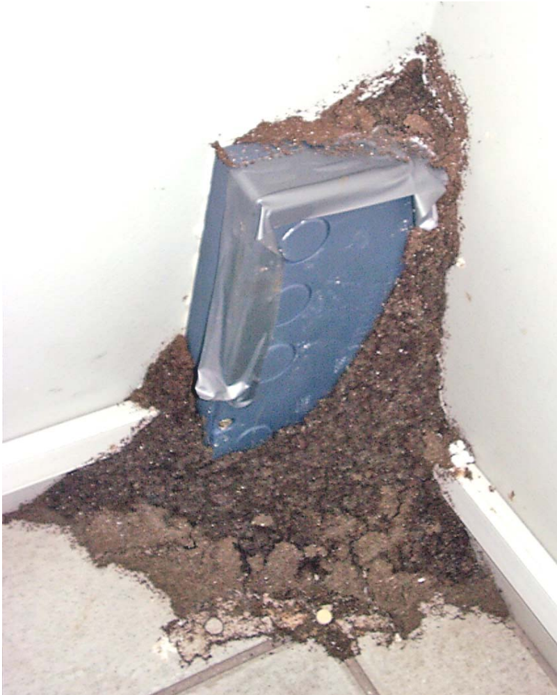
Termite workings encasing an AG Station.
