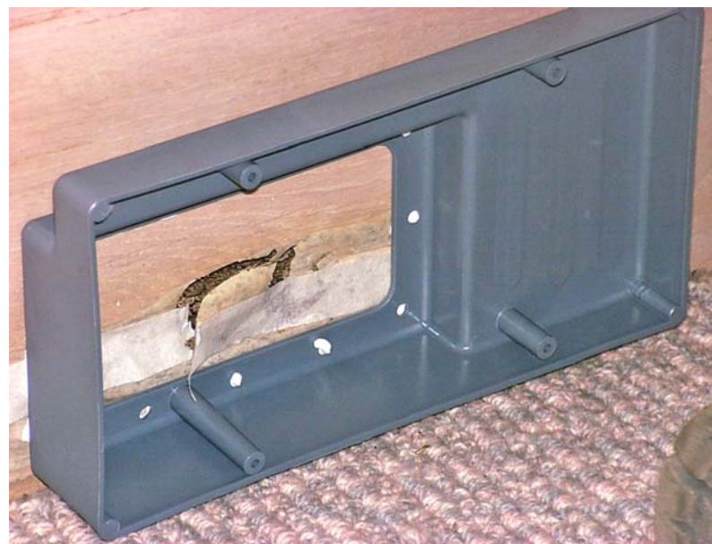
Above-ground Station being installed over termite damaged timber.
