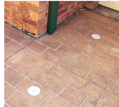
IC Stations sealed with stainless steel caps.
