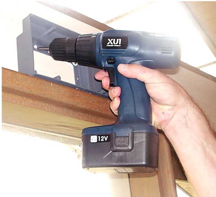
Affixing an AG Station to a wall above a door frame.
