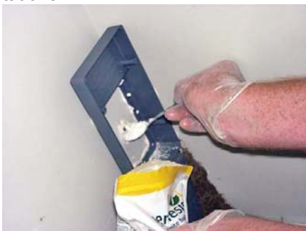
Applying NEMESIS bait by spoon directly to the termite workings.
