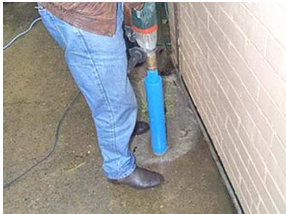
Using concrete coring drill for station placement.
