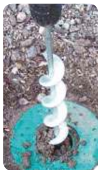
Picture 6: Cordless drill with auger attachment for cleaning out IG Stations.
