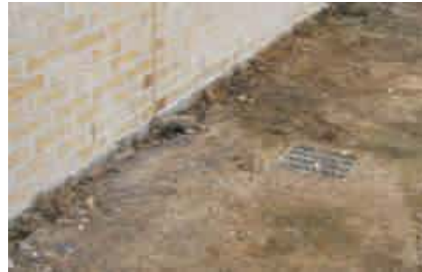
Note drain adjacent to building
