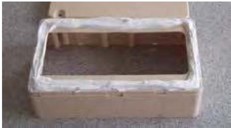
Photo 1. Selleys No More Gaps spread on the base of the AG station.
