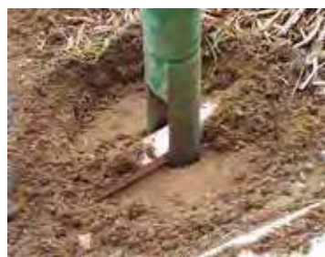
Photo 4. A piece of wood in the auger channel helps clear the soil surface to create a flat base for the Sentricon station. It may also be used to clear lawn, gravel or mulch.
