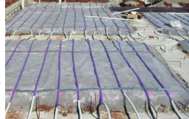
Source: Altis Anti Termite Irrigation System - 2017 Version 5
